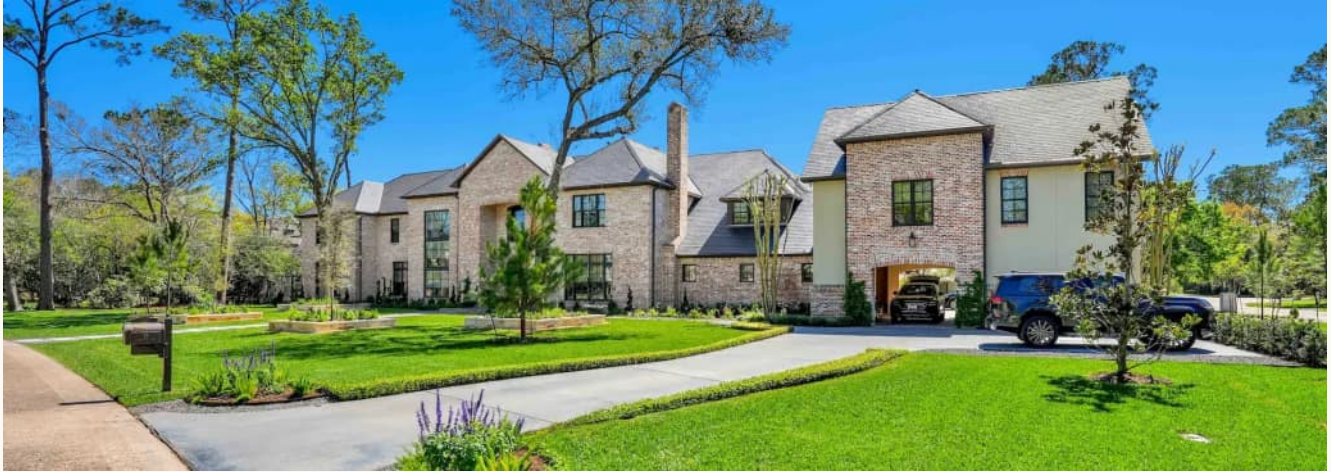
PHOTOGRAPH — THE PROPERTY AS BUILT
